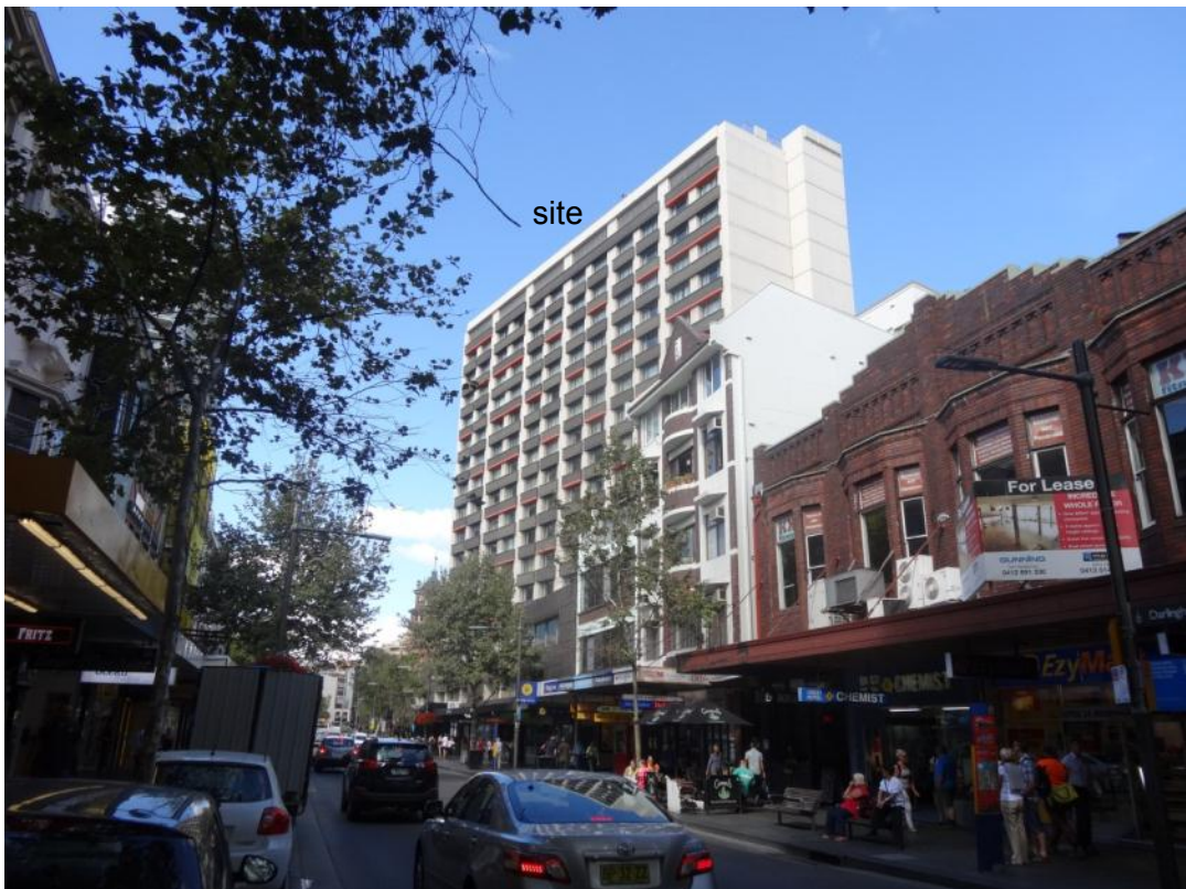
Figure 5: View of the site looking south west along Darlinghurst Road
