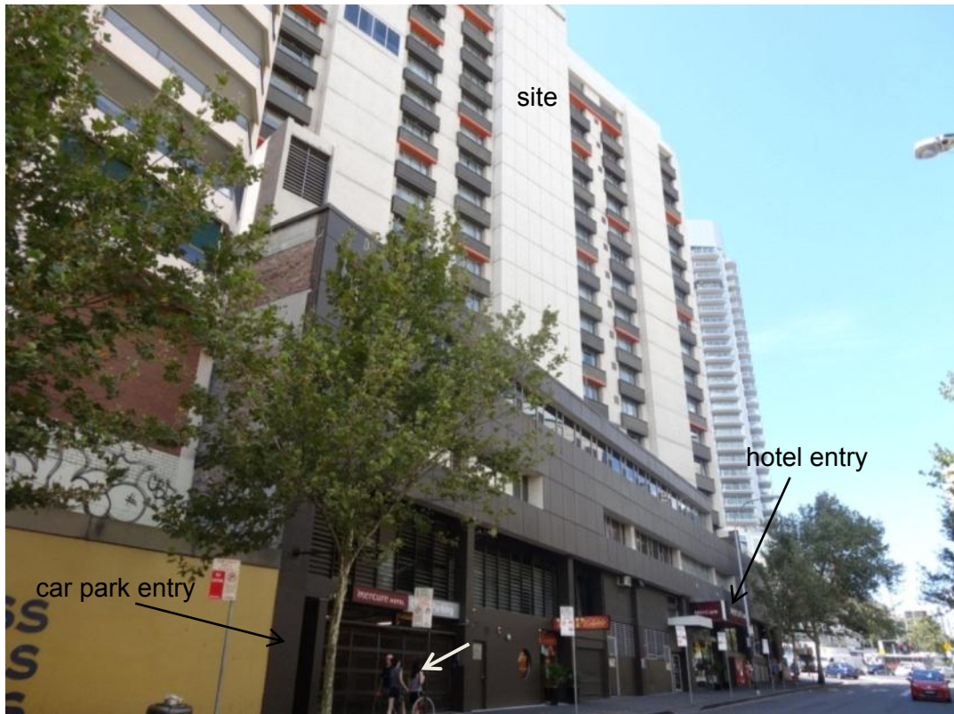
Figure 6: View of the western facade of the site addressing Victoria Street, with a 3 storey podium containing entries to the car park and hotel foyer and a substation.
