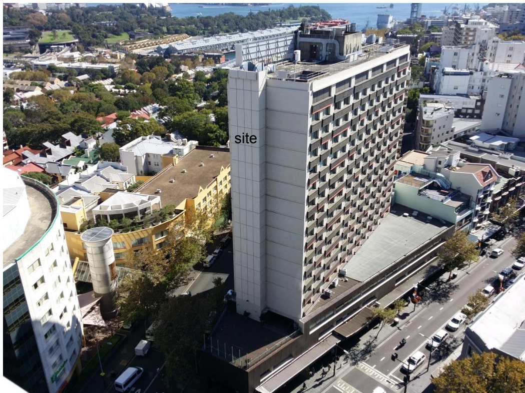
Figure 3: View of the site from adjacent residential tower located to the south, showing the plant room, wind breaks and associated services located on the roof
